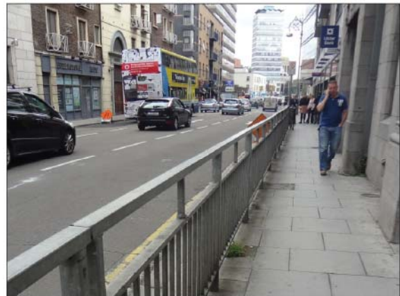
Figure 2.10: Guardrails can create a hazard for cyclists, reduce footpath widths and give rise to feelings of constraint and restriction to pedestrians.
