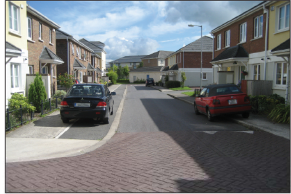
Figure 2.12: If on-street parking is not provided, particularly for visitors, it can lead to poor parking behaviour from drivers who kerb mount and park on footpaths/cycle lanes.
