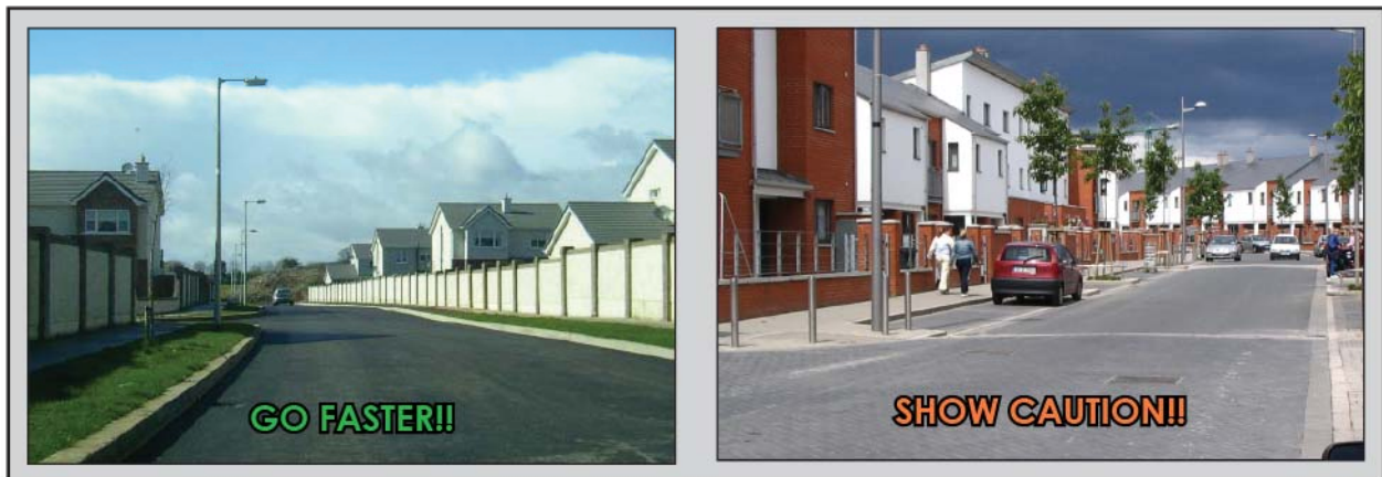
Figure 2.14. The elimination of access and frontage along roads (top) was introduced to reduce risk, but it serves to encourage speeding.
