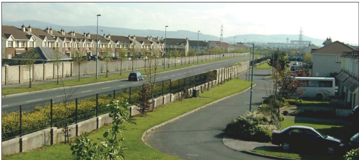
Figure 2.6: Distributor Road which creates severance between communities. The road is designed to minimise any disruption to vehicle movement by restricting the number of junctions and pedestrian access (through the use of walls and fences). The road is also frontage free, eliminating the need for driveway access to individual properties.
