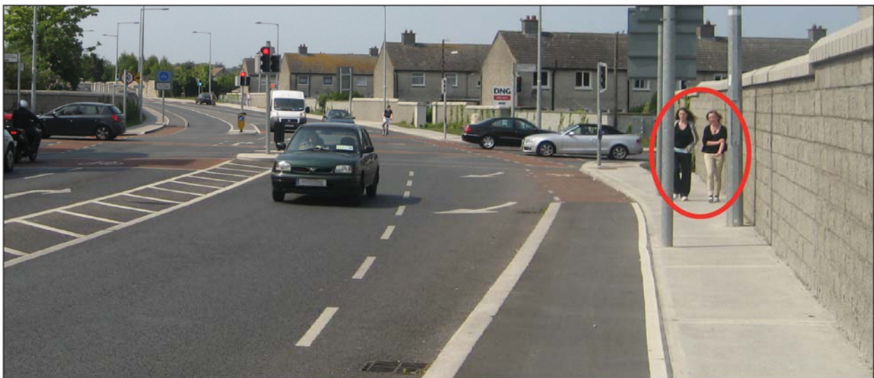
Figure 2.11: Pedestrians have been marginalised along the street edge and have their path obstructed in order to provide additional width to the vehicular carriageway and space for signage.
