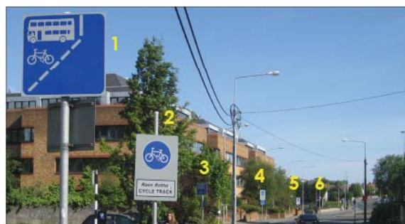
Figure 2.17: Examples of updesigning which provide little cost benefit. From top to bottom, large splayed junction, complex junctions, ramps on wide carriageways, noise walls and repetitive signage.
