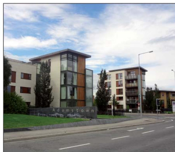
Figure 3.17: Example of a Gateway from Adamstown, Co. Dublin, where changes to the built form and landscaping treatments add to the sense of enclosure and create a formal entry point.
