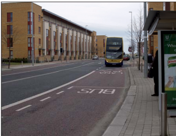
Figure 3.28: QBCs and Bus lanes should be considered on all Strategic Routes where the high frequency services occur or where their future need has been established.
