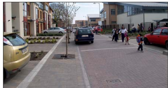
Figure 3.20: Examples from Adamstown, Co. Dublin. Through routes (top) are designed to cater for more moderate speeds and to prioritise public transport movement. Local streets (bottom) are slower moving, thus discouraging use by through traffic.
