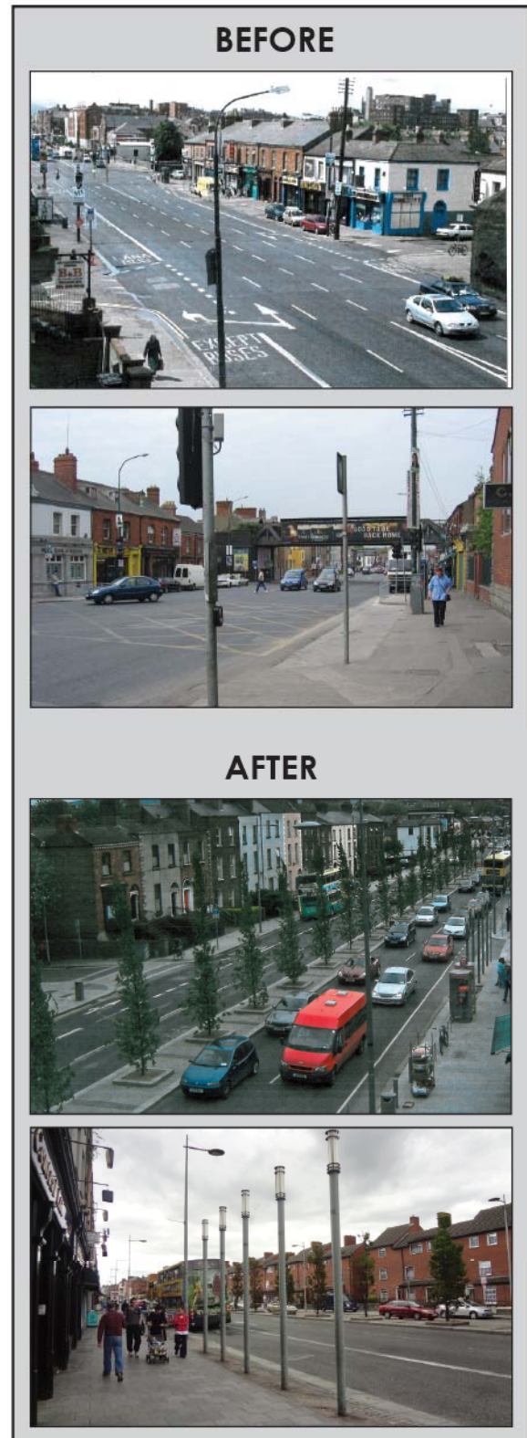
Figure 5.1: Images of Dorset Street, Dublin (part of the N1 national route), demonstrate how better outcomes can be achieved by shifting away from convention and embracing a more inclusive and strategic approach to design.
