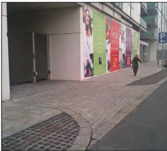
Figure 4.35: Example from Dublin where pedestrian priority across driveways is indicated by maintaining footway levels and surface treatments.
