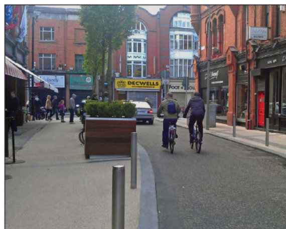
Figure 4.26: Fade Street, Dublin City Centre. To reduce the overall cost of work in remodelling the street, lower budget materials such as HRA with coloured aggregate chips and epoxy resin bound surfaces were used on the carriageway and footpath, respectively.
