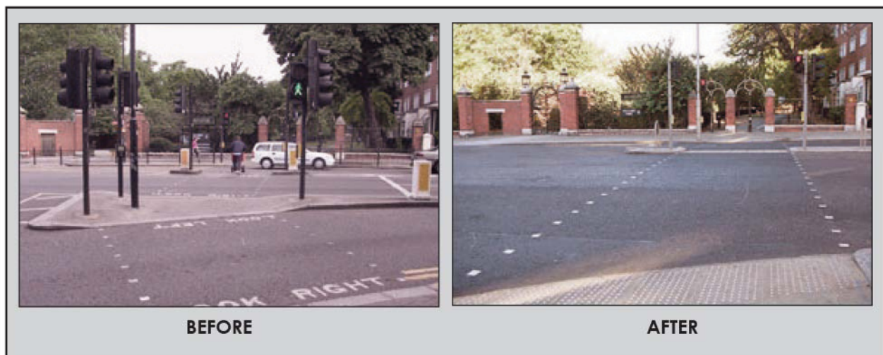
Figure 4.40: Example from Kensington High Street, London, of a left hand turning slip point was removed and replaced with a safer single phase crossing which also slowed vehicle turning movements (image source: Hamilton Baillie).
