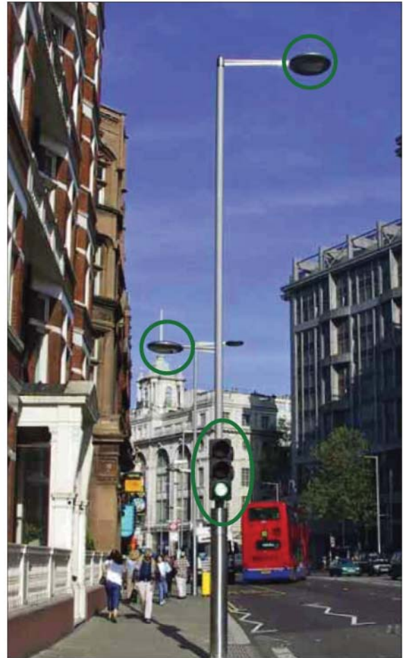
Figure 4.22: Example of a light installation that is designed with both the pedestrian and the vehicle in mind and also incorporates signals for a pedestrian crossing (image source: Camden Streetscape Manual).
