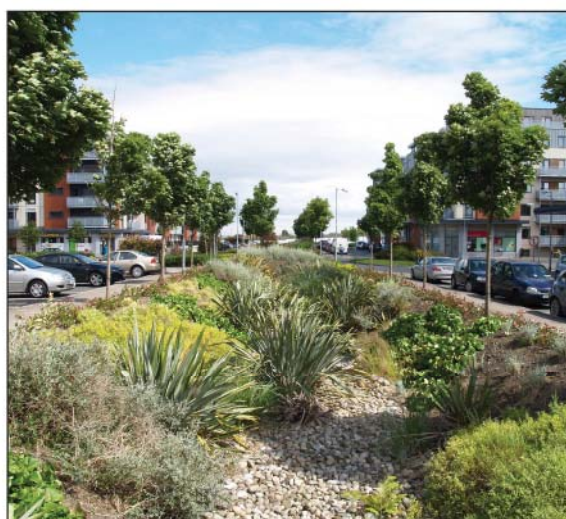
Figure 4.29: Examples of Sustainable Urban Drainage incorporated into a street in the form of a small 'swale' (top) and larger linear basin (bottom). These treatments not only assist in containing urban surface water run-off but also contribute to the sense of place by adding a unique feature.
