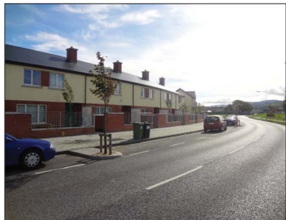
Figure 4.77: Example from Fettercairn, Co. Dublin where a 'distributor' style road was narrowed by adding bays of parallel parking as part of a package of works aimed at calming traffic and improving the sense of place.
