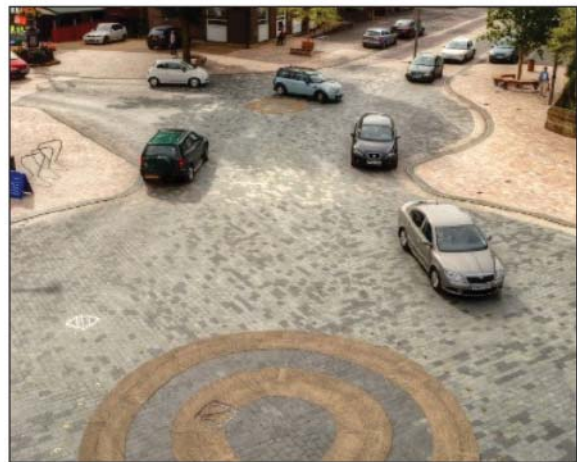
Figure 4.61: Examples from Ashford, UK (top) and Poynton, UK (bottom). The placement of a circular features with the shared space/traffic calmed environment creates an informal roundabout with fewer restrictions pedestrian/cyclist movement when compared to more conventional types (image sources: Hamilton-Baillie Associates and Ashford Borough Council).
