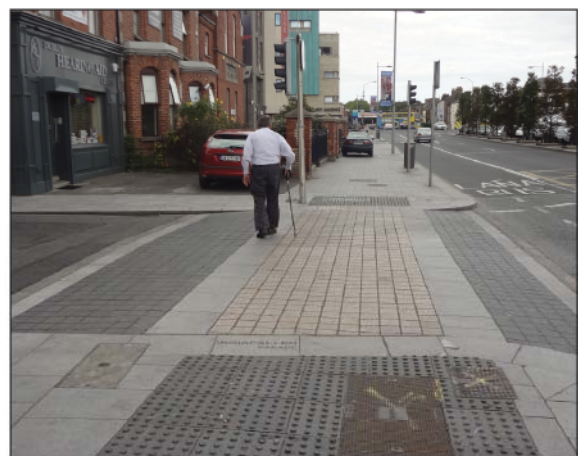
Figure 4.69: Example from Dorset Street, Dublin, where the carriageway has been raised and paved to slow turning vehicles and enhance the pedestrian crossing.
