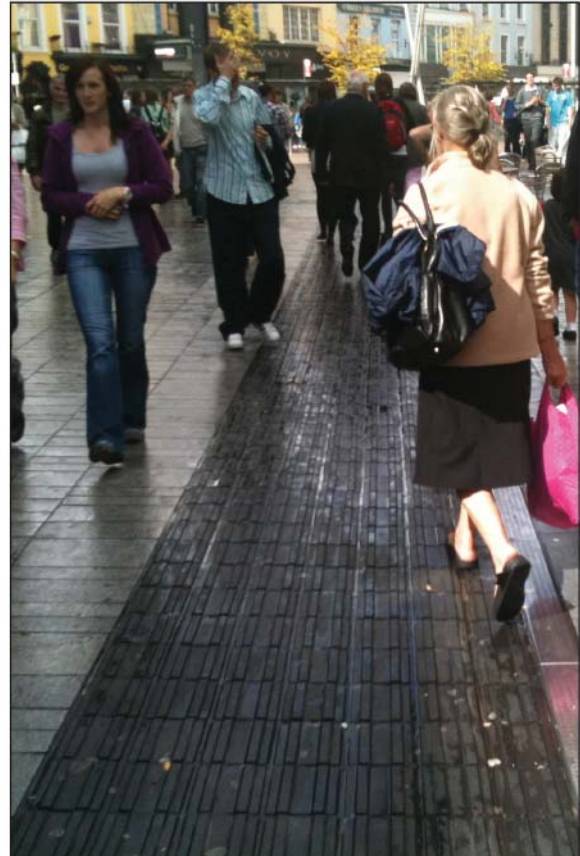
Figure 4.50: Examples from Cork city of the use of tactile paving that assist the visually impaired by guiding movement across a shared space.
