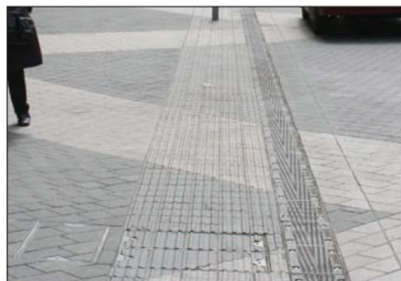
Figure 4.74: Example of a drainage channel on Exhibition Road, London. The kerb line indicates an area of pedestrian refuge and is used to guide the visually impaired.
