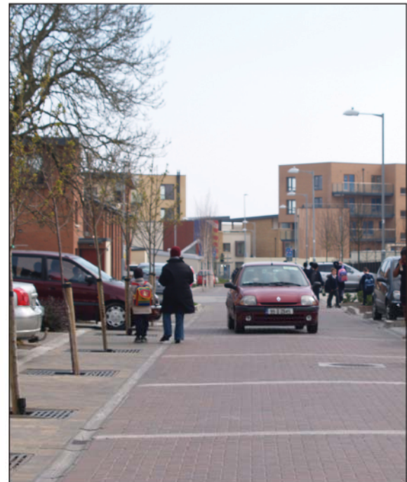
Figure 4.51: Examples from Adamstown, Co. Dublin, where a verge is provided as refuge that pedestrians can hop on and hop off as cars slowly pass.
