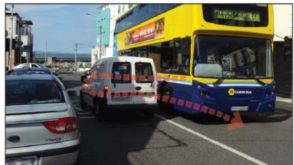
Figure 4.45: Setback stop lines allow for additional vehicular manoeuvrability for larger vehicles at signalised junctions without the need for larger corner radii.
