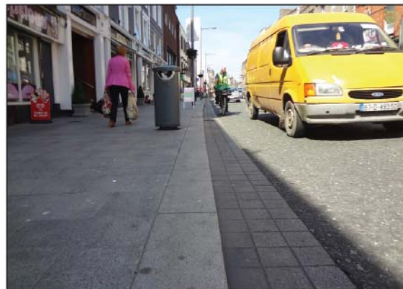
Figure 4.72: Example of a low kerb from Drogheda, Co. Louth, which is used to reinforce lower design speeds and create a greater sense of shared space.
