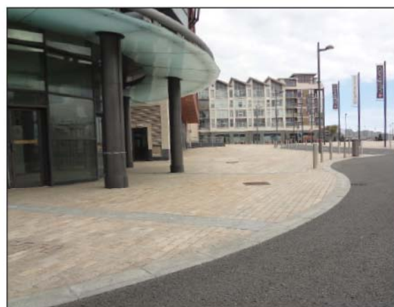
Figure 4.73: Example from Clongriffin Co. Dublin, where the footpath, kerb line and vehicular carriageway are at the same level. Whilst pedestrian and vehicular space are still clearly defined, a greater sense of shared space is still created.
