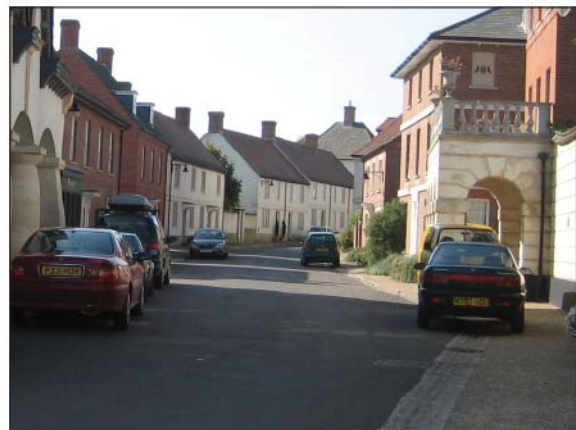
Figure 4.70: Examples from Poundbury, Dorchester, UK, where changes in the kerb line and carriageway alignment calm traffic by limiting forward visibility, creating pinch points and requiring multiple changes in direction.
