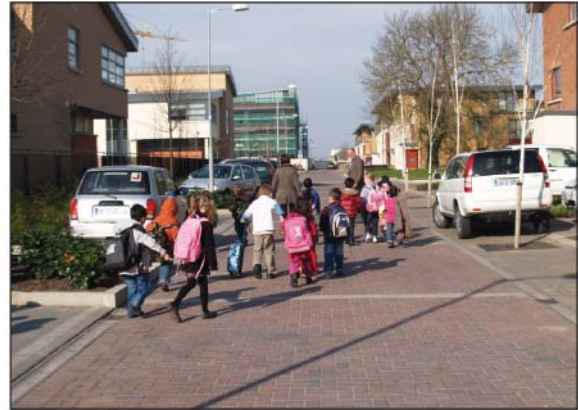
Figure 4.56: Example from Adamstown, Co. Dublin of a shared surface 'homezone' adjacent to a school. Paving materials, combined with embedded kerbs encourage a low speed shared environment.
