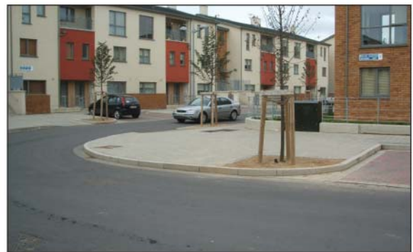
Figure 4.75. Example from Ballymun, Co. Dublin (top) and Leixlip, Co. Kildare (bottom) where kerb build-outs and contrasting materials are used to separate and define bays of parking from the vehicular carriageway, reduce corner radii and facilitate planting or landscape treatments.
