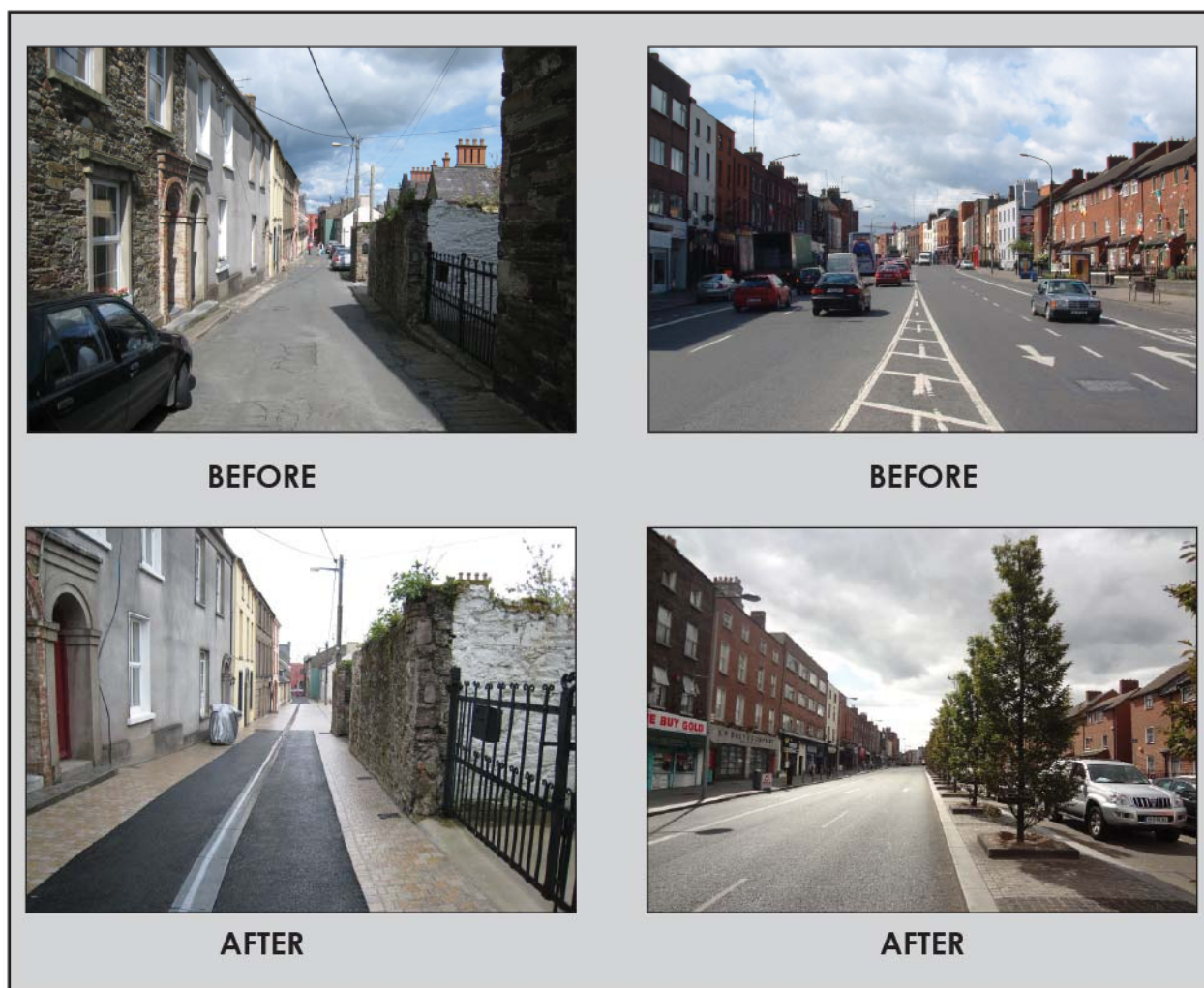
Figure 4.6: Examples from Youghal, Co. Cork (left), and Dorset Street, Dublin City (right), of retrofitted design responses that are appropriate according to Context and Function. The narrow, enclosed and lightly trafficked nature of the street within Youghal is highly suited to a shared carriageway. The heavily trafficked nature of Dorset Street makes it highly suited to a Boulevard type configuration.
