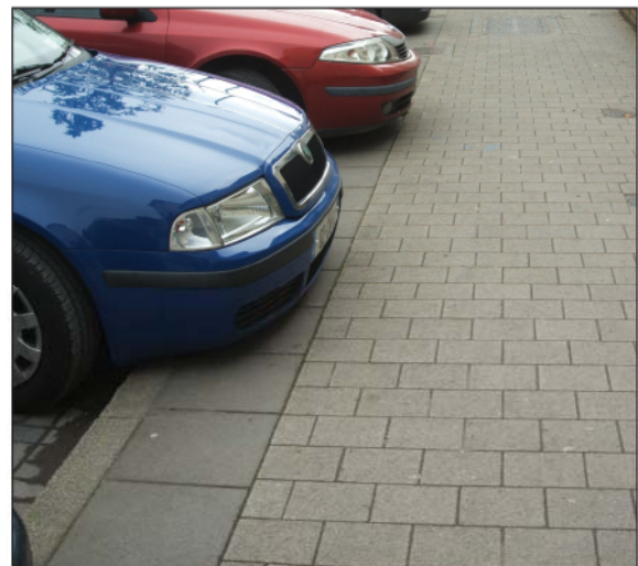
Figure 4.36: An example where a narrow verge is provided to ensure that vehicle overhangs do not intrude on the footway.
