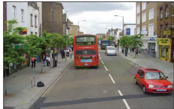
Figure 4.15: Walworth Road, Central London, UK, before (top) and after (bottom). The street carries over 20,000 vehicles per day and as part of major upgrade signage and line marking were minimised (image source: Southwark Council).
