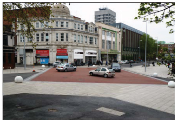
Figure 4.62: Example from Coventry, UK of a shared surface uncontrolled junction. The level of traffic using the junction would normally warrant some form of control, however, its traffic calmed nature allows for drivers to communicate with each other and pedestrians to establish movement priorities (image source: Hamilton-Baillie Associates).
